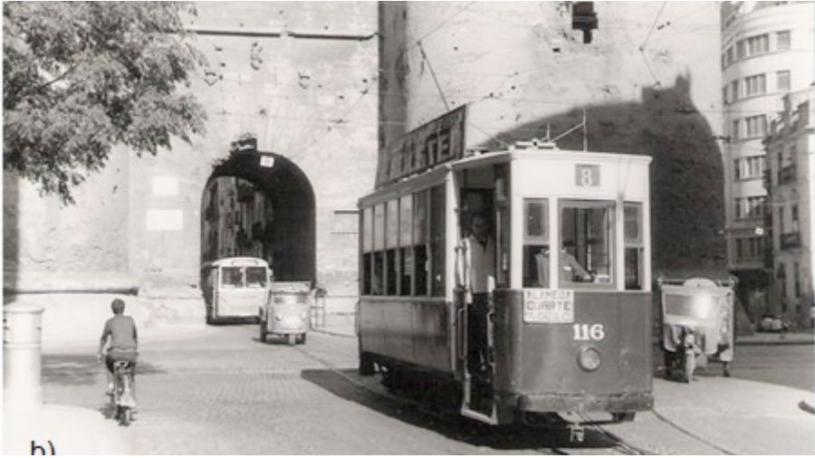
Figure 1.8b. Photograph of a tram 116 serving the line 8: “Alameda-Cuarte-Fernando el Católico” after passing under the mediaeval Cuarte towers. This tram line was operative between 1 st July 1964 and 7th October 1965. Col. Solaz Albert.
