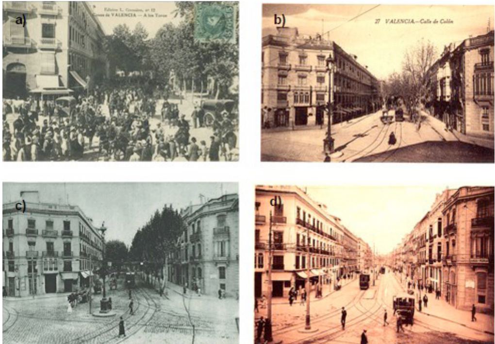
Figure 1.10a-d. Four images of the intersection between the Ruzafa , Xàtiva and Colón streets in Valencia from postal cards of the Cols. Huguet and Solaz Albert. a) Postal card circulated in 1901 showing a horse streetcar of the Diagonal line in its starting point, and b-d) three images of the electrified period before 1930. See text for chronological information.
